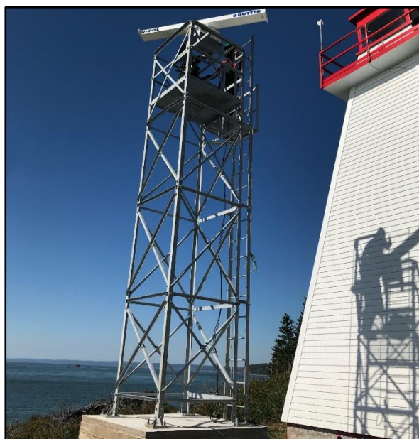
Figure 3: One of two high-resolution radars constructed near the FORCE site to be used for the Risk Assessment Program.
